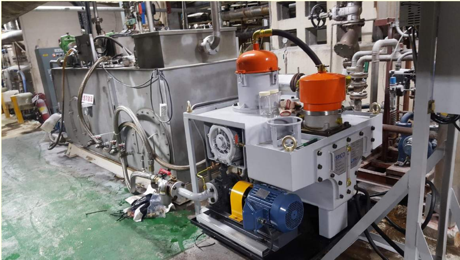
GP200 Installation(Sludge and water separator)
