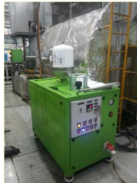
Sam lak Heat treatment PCC602 installation
