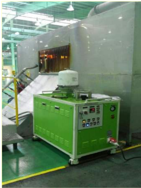
ILJIN Bearing art PCC602 installation
